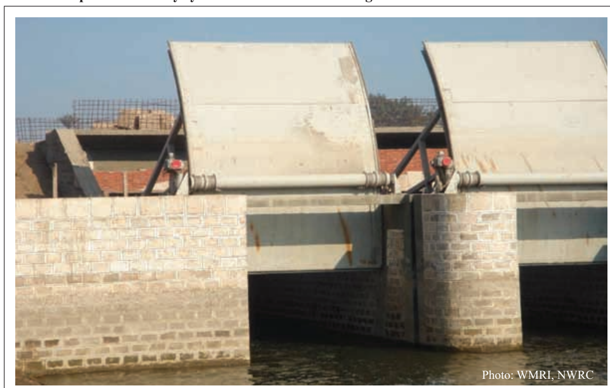
Photo 2: Improved Delivery system: Radial Gates on Irrigation Offtake
