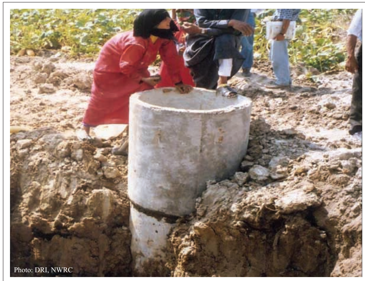
Photo 3: Installation of Pre-Cast Concrete Manholes
