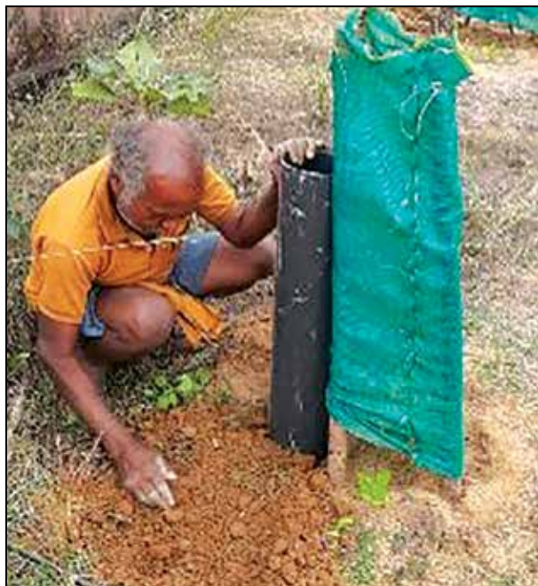
Figure 28. Fixing of sub-surface irrigation and tree guard
