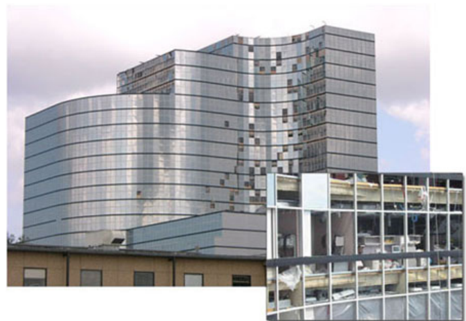
Figure 4. Information about secondary risk modifiers, such as the percentage of glass in a building envelope, can be very significant for accurately estimating losses. Source: AIR
